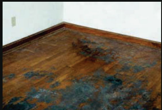
Water or pet stains (pet stains may not come out even after total resanding).
